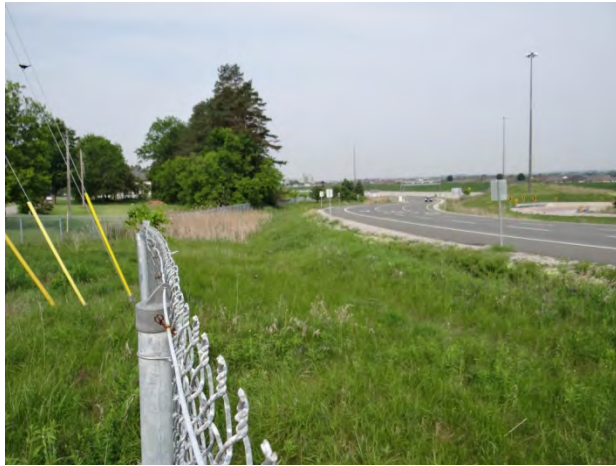
Plate 3: Study area west of McCowan Road, looking west.
